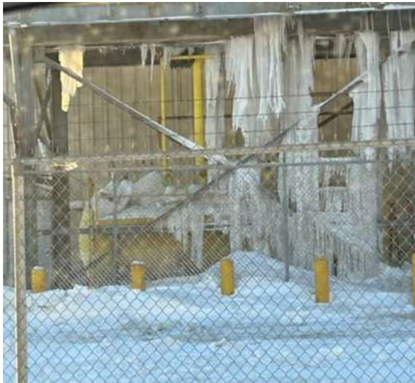
Figure 7. Ice Buildup Near the High Pressure Receiver
