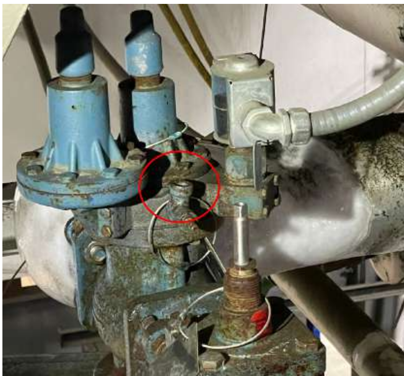
Figure 26. Service Valve Left Open to Atmosphere
