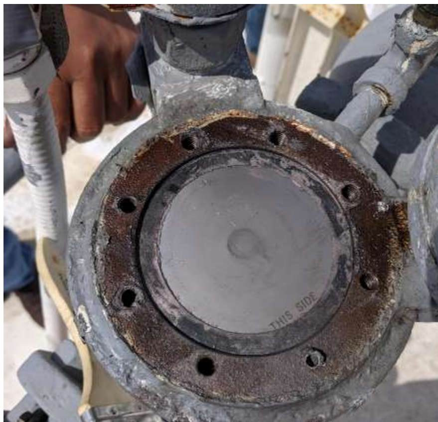
Figure 28. Partially Disassembled Suction Regulator
