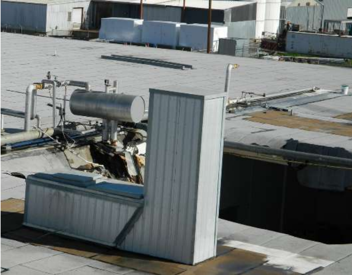
Figure 1. Collapsed Roof Viewed from Above
