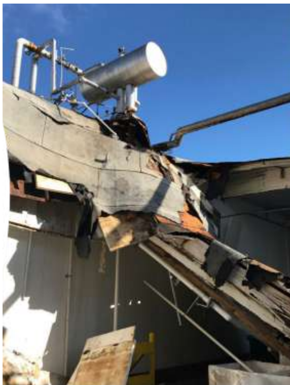
Figure 2. Collapsed Roof Viewed from Below
