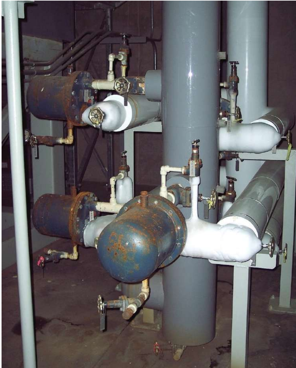
Figure 11. Vessel-to-vessel float assembly.
