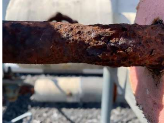
Figure 10. Swelling rust/corrosion.
