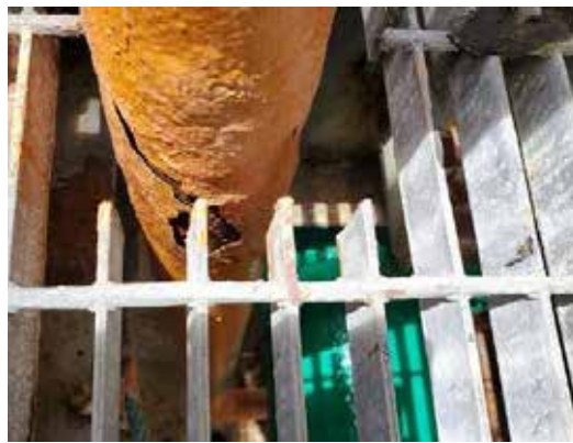
Figure 8. Blister rust/corrosion.
