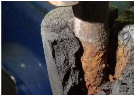
Figure 6. Elastomeric foam insulation on ammonia piping.
