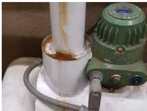
Figure 5. Water pooling at the base of insulated ammonia piping at pump out.
