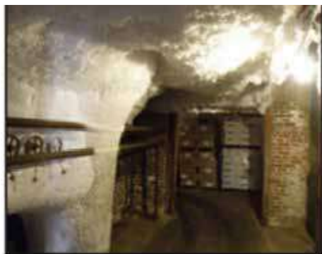
EPA inspection photo reveals dangerous ice buildup on ammonia piping and valves.
