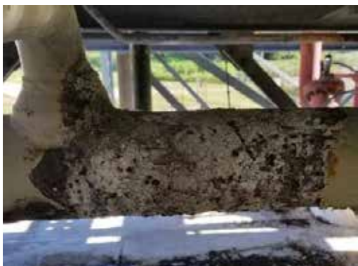
Figure 4. Chemically induced corrosion on bare piping.
