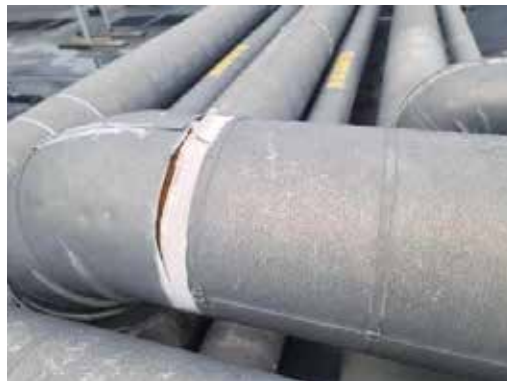
Figure 3. Jacketing separation and split seam
