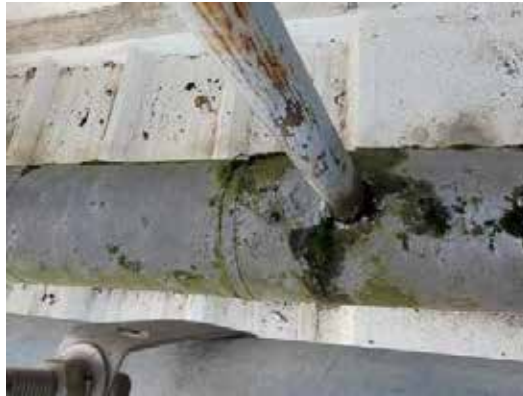
Figure 7. Algae on the ammonia pipe jacketing.
