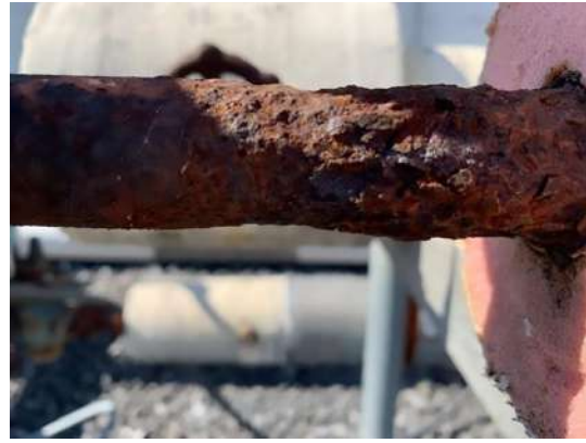
Figure 10. Swelling rust/corrosion.
