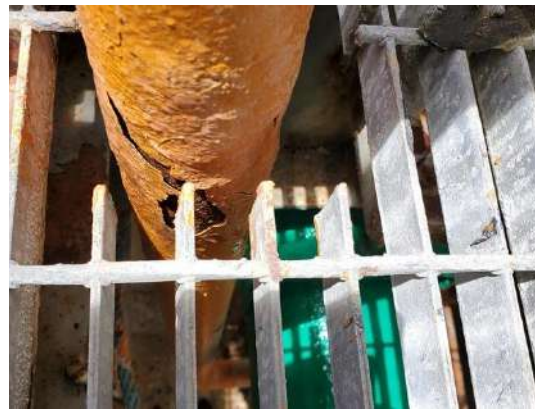
Figure 8. Blister rust/corrosion.
