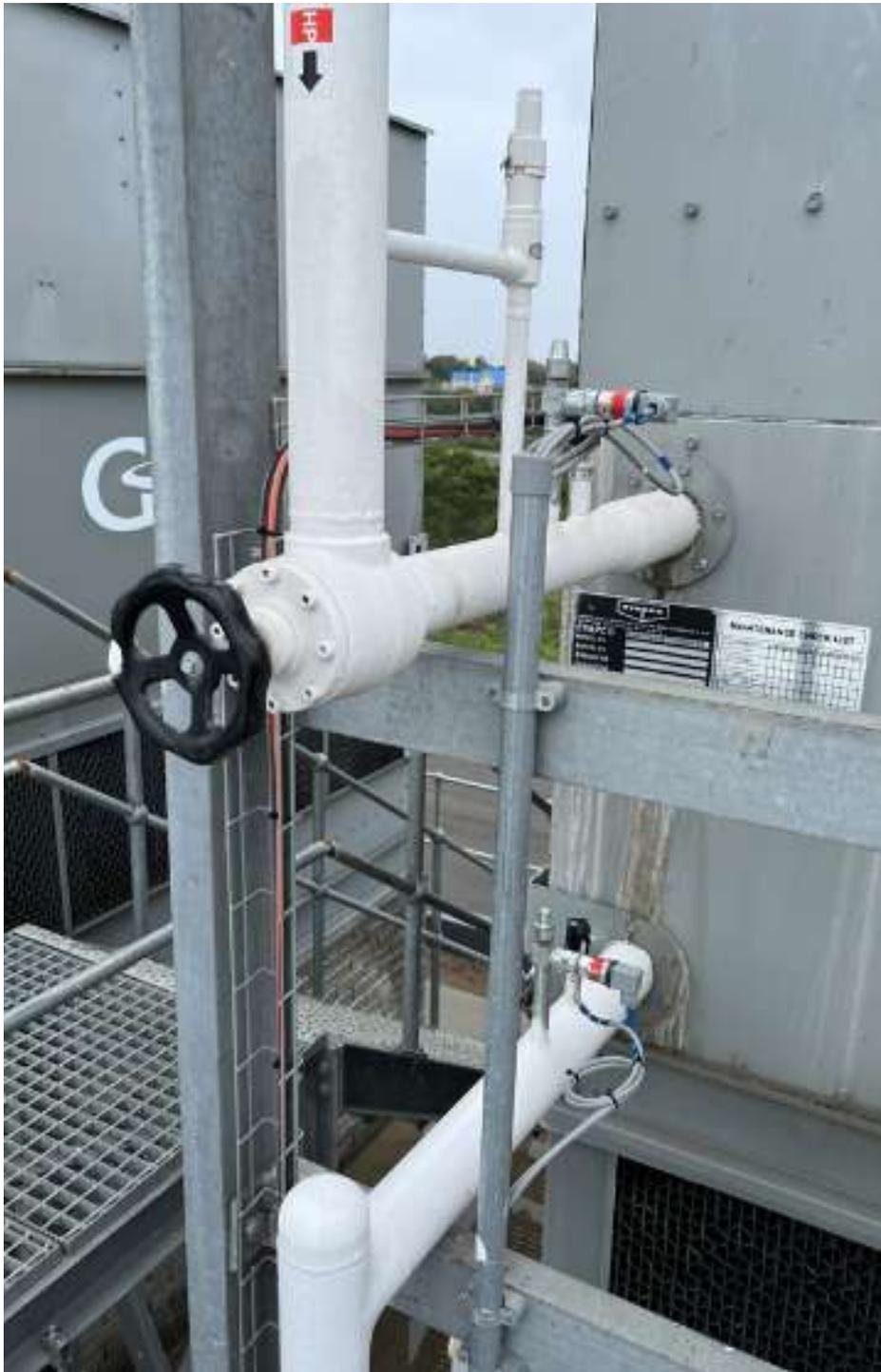
Figure 17. The pressure and temperature sensors used for taking measurements.
