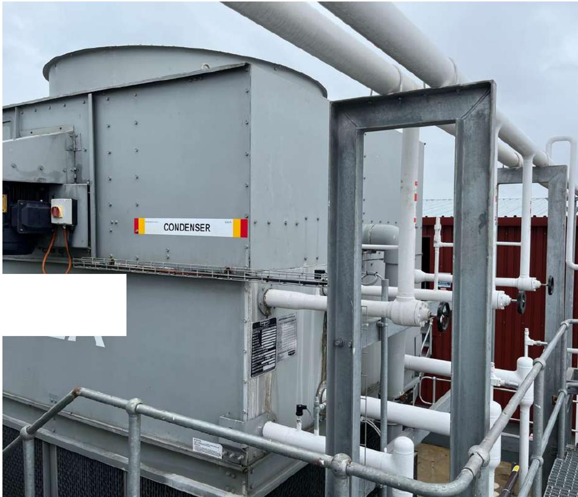
Figures 16. The additional circuit on the evaporative condenser for the de-superheating coil.
