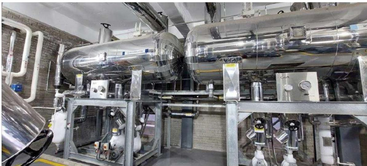
Figure 14. Machinery room with a view of the separator vessels.
