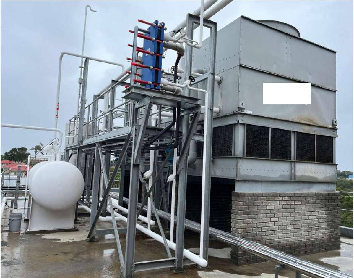
Figure 15. Evaporative condensers, liquid receiver, and heat recovery condenser.
