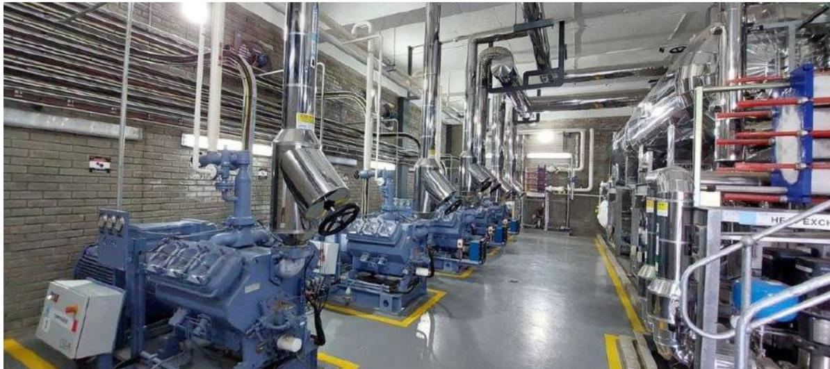
Figure 13. Machinery room with a view of the high-stage and low-stage compressors.
