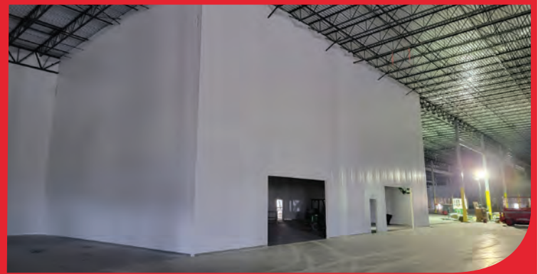
Box in Box
