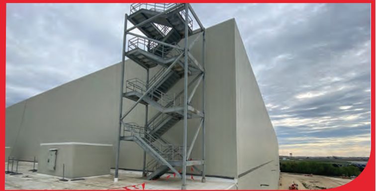
Full Building Construction
