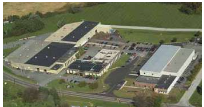
GEA Heating & Refrigeration Technologies – North America York, Pennsylvania
